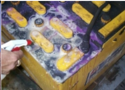
Fig. 1 An example of a poorly maintained battery. This battery will require more charge time and, as a result, less work time.
